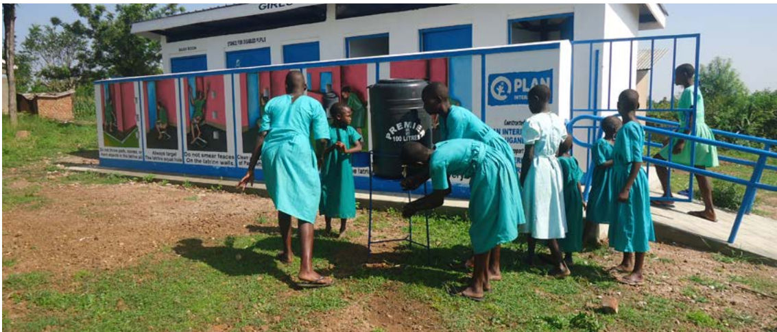
A latrine facility at Abia Primary School in Kamuli District clearly showing the toilet use instructions
